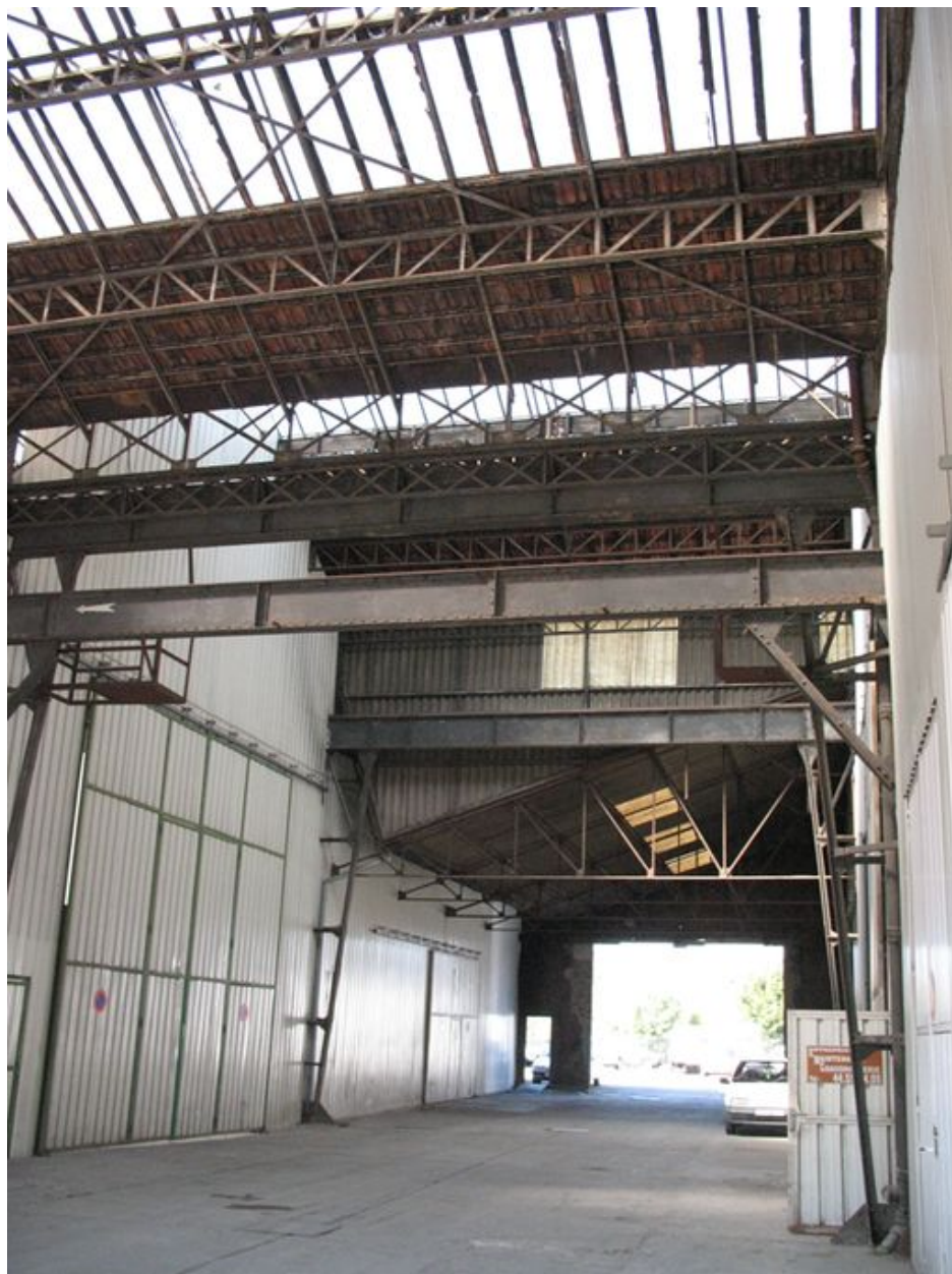
Structures des charpentes.
