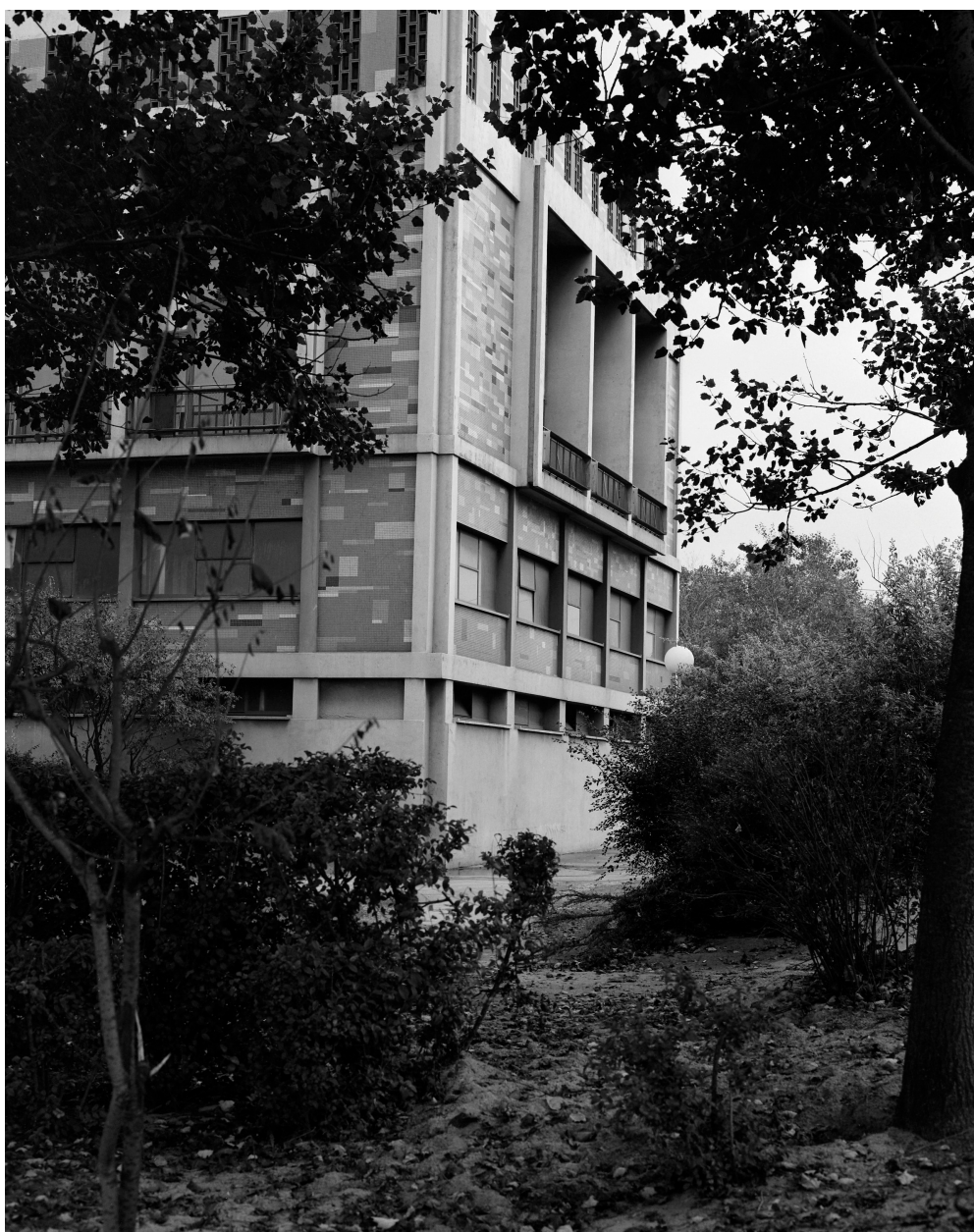
Casino municipal, pignon sud.
