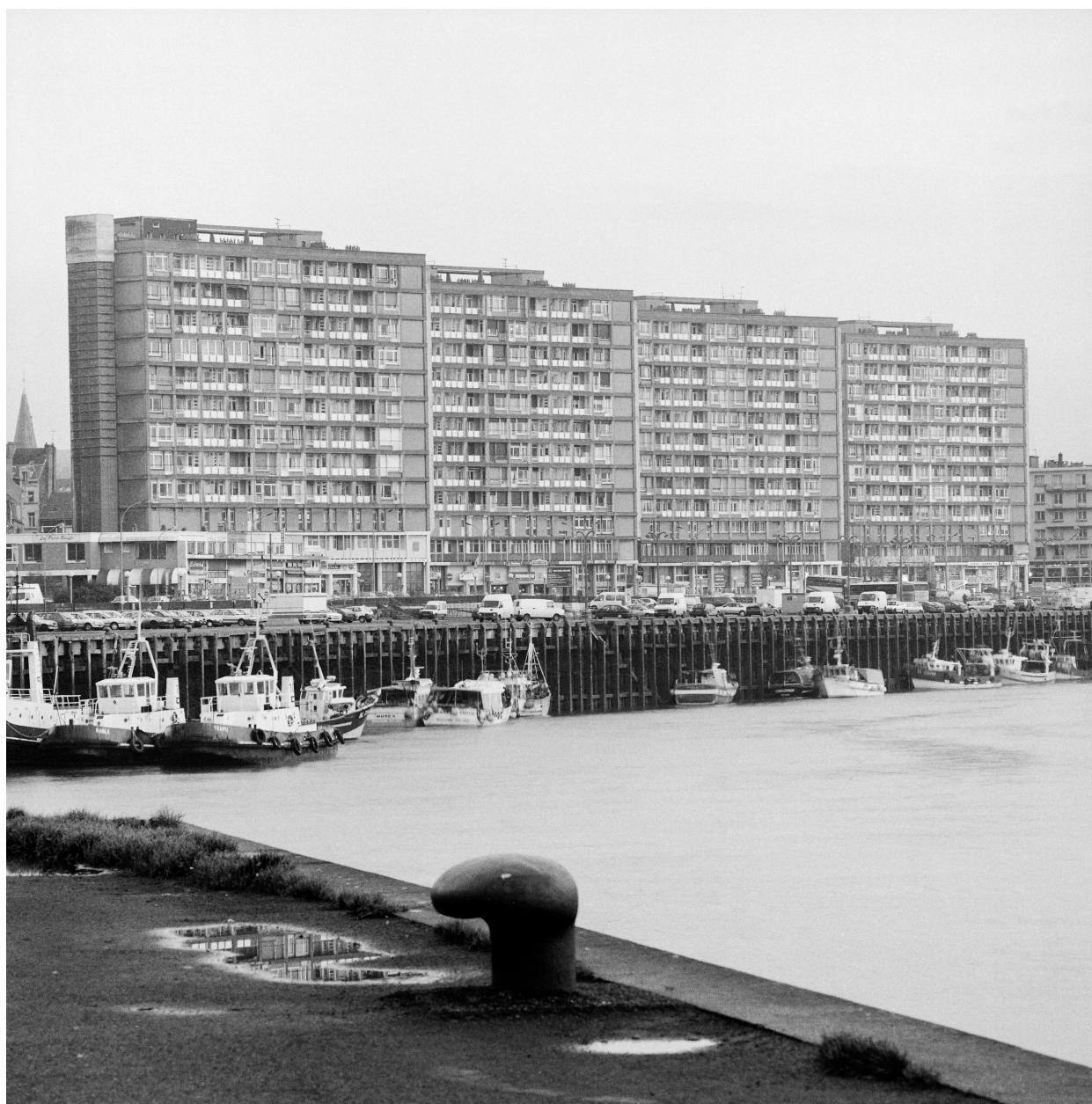
Reconstruction immeubles dits buildings A B C D, boulevard Gambetta.
