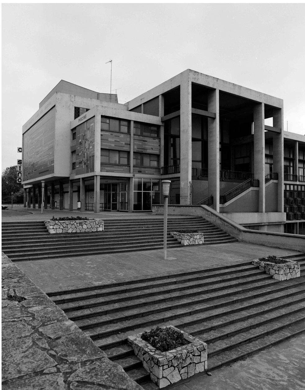
Casino municipal, angle nord.
