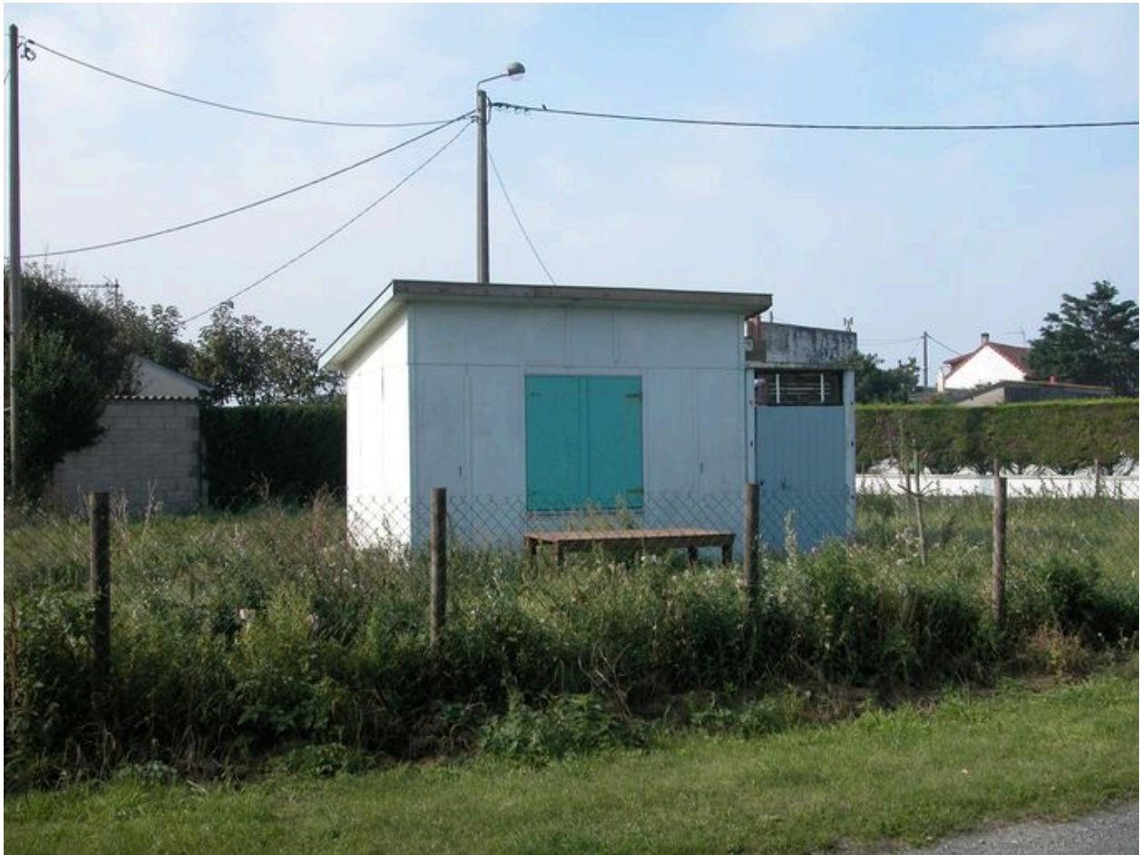
Bungalow, rue de Bougainville (1988 AY 175).
