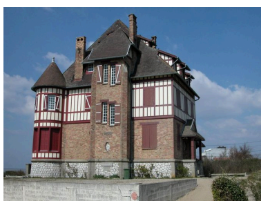
Elévation sud-est. Phot. Elisabeth Justome IVR22_20048001609NUCA
