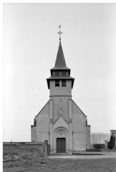
Elévation occidentale. Phot. Jean-Michel Perrin IVR22_19856000005X
