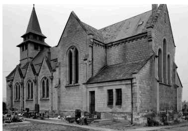
Elévation sud. Phot. Jean-Michel Perrin IVR22_19856000006X
