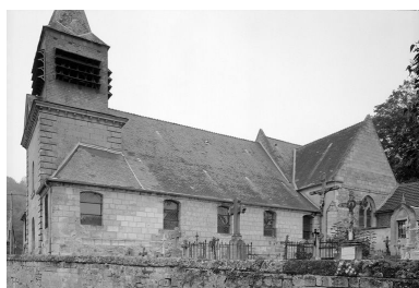
Elévation sud. Phot. Jean-Michel Perrin IVR22_19846001207X
