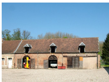
Remises agricoles. Phot. Frédéric Fournis IVR22_20118001280NUCA
