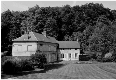
Logement patronal, angle sud-est. Phot. Patrick Glotain IVR22_19936000566X
