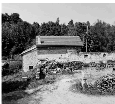
Remise. Phot. Patrick Glotain IVR22_19936000569X
