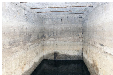
Salle S5 Phot. Pierre Thibaut IVR31_20155901424NUCA
