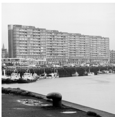
Reconstruction immeubles dits buildings A B C D, boulevard Gambetta. Phot. Philippe Dapvril IVR31_19946200768X
