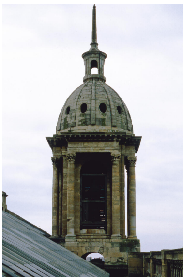
Basilique, tour nord, façade est. Phot. Jean-Michel Périn IVR31_19876201476ZA
