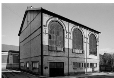
Chaufferie, flanc sud. Phot. Francis Dubuc IVR22_19908001105Z
