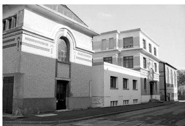
Bureau, chaufferie. Phot. Francis Dubuc IVR22_19908001110Z
