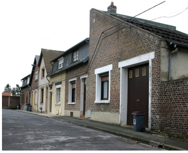
Façade antérieure. Phot. Frédéric Pillet IVR22_20060205039NUCA
