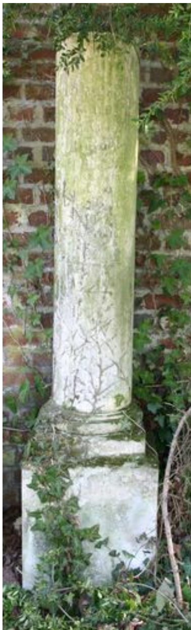
Colonne. Phot. Caroline Vincent IVR22_20068000954NUCA
