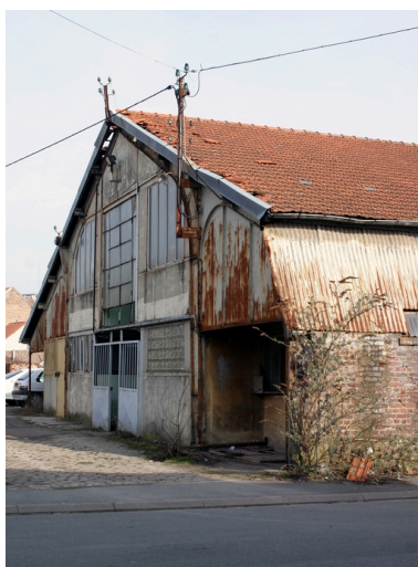
Magasin industriel. Phot. Frédéric Pillet IVR22_20050205294NUCA
