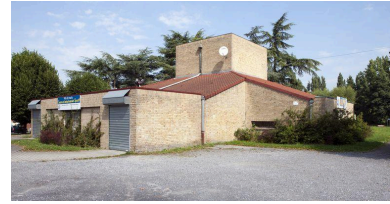
Élévation sud est. Phot. Pierre Thibaut IVR31_20155900718NUCA
