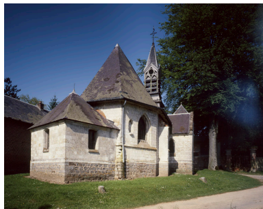
Eglise Saint-Antoine. Phot. Irwin Leullier IVR22_19988000582VA
