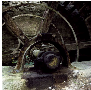
Roue hydraulique verticale. Phot. Olivier Coquelle IVR22_19946000940XA
