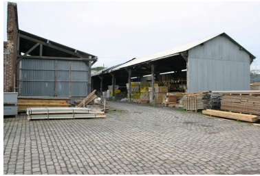
Hangars. Phot. Frédéric Pillet IVR22_20070205068NUCA
