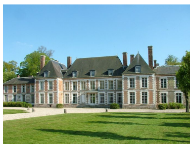
Corps de logis principal. Phot. Frédéric Fournis IVR22_20118001253NUCA
