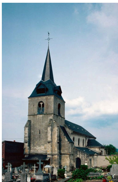
Façade occidentale. Phot. Michel Hérold IVR22_19856000934ZA
