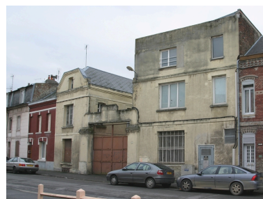
Façade antérieure. Phot. Frédéric Pillet IVR22_20070205089NUCA
