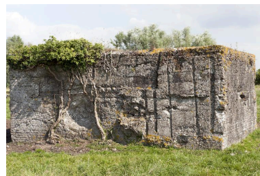
Elévation nord. Phot. Jean-Marc Ramette IVR31_20145905363NUCA
