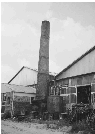
Atelier de fabrication, flanc est. Phot. Benoît Dufournier IVR22_19936001622Z
