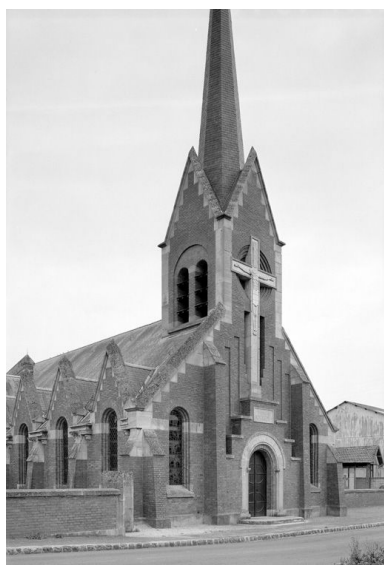
Façade occidentale. Phot. Jean-Michel Perrin IVR22_19846001076X
