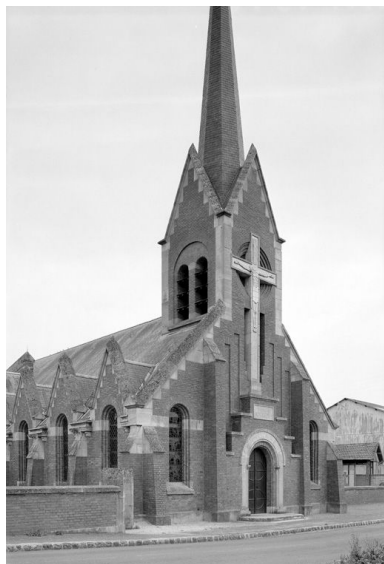
Façade occidentale. Phot. Jean-Michel Perrin IVR22_19846001076X
