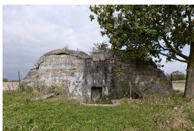
Elévation sud Phot. Jean-Marc Ramette IVR31_20155904747NUCA
