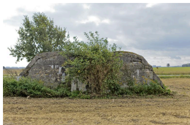
Pignon nord Phot. Jean-Marc Ramette IVR31_20155904753NUCA
