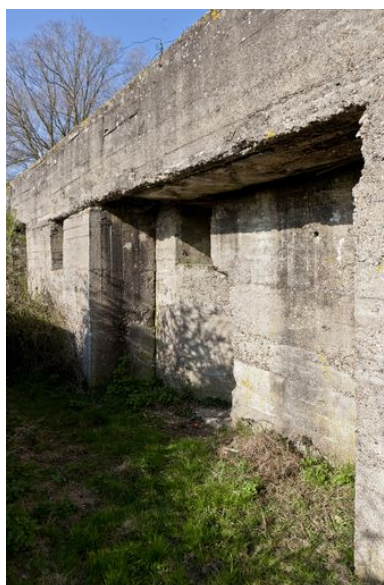
Elévation sud. Phot. Jean-Marc Ramette IVR31_20145905406NUCA
