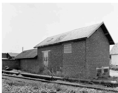
Station de pompage. Phot. Patrick Glotain IVR22_19936000756X
