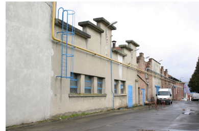
Pignons orientaux des ateliers. Phot. Frédéric Pillet IVR22_20060205243NUCA
