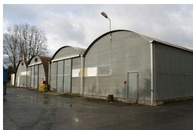
Hangars. Phot. Frédéric Pillet IVR22_20060205253NUCA
