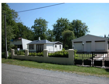
Maisons (50, 52, 54 avenue des Sapins, AE 47, 48, 49). Phot. Elisabeth Justome IVR22_20058004003NUCA
