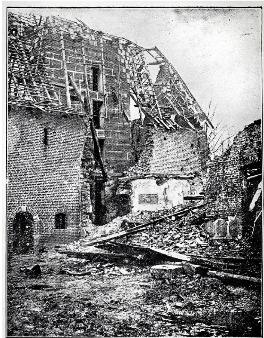
18.—SOMERSET FARM. VIEW OF THE O.P. TOWER FROM THE COURT-YARD.
