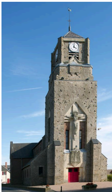
Façade principale est. Phot. Marie-Laure Monnehay-Vulliet IVR32_20188000601NUC2A
