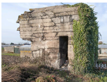
Elévation sud Phot. Jean-Marc Ramette IVR31_20145904957NUCA
