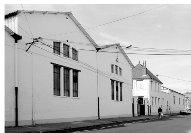
Vue partielle, flanc est. Phot. Francis Dubuc IVR22_19908000972Z
