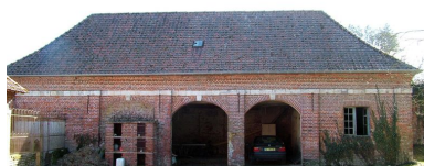
Remise agricole (?). Phot. Frédéric Fournis IVR22_20108001146NUCA
