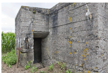
Elévation sud Phot. Jean-Marc Ramette IVR31_20145905476NUCA
