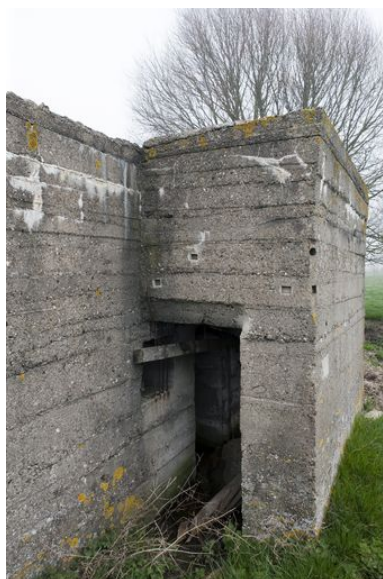
Elévation sud, porche pare-souffle Phot. Jean-Marc Ramette IVR31_20145905485NUCA
