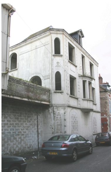
Le logement patronal. Phot. Frédéric Pillet IVR22_20070205082NUCA
