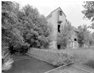
Elévation ouest. Phot. Patrick Glotain IVR22_19898000160V
