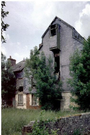
Elévation ouest. Phot. Patrick Glotain IVR22_19898000240XA
