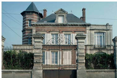
Elévation antérieure. Phot. Alain Nafilyan IVR22_19856001323ZA
