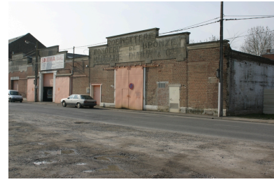
Les ateliers subsistants, quai Gayant. Phot. Frédéric Pillet IVR22_20050206195NUCA
