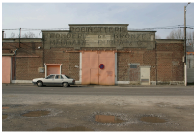
Atelier, quai Gayant. Phot. Frédéric Pillet IVR22_20050206196NUCA
