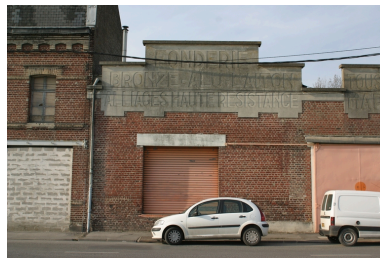
Atelier, quai Gayant. Phot. Frédéric Pillet IVR22_20050206197NUCA
