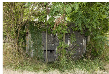
Elévation nord Phot. Jean-Marc Ramette IVR31_20145905182NUCA
