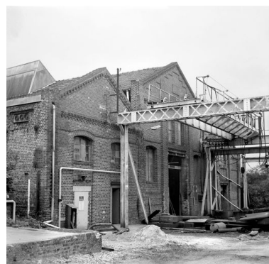
Atelier de fabrication 1, flanc ouest. Phot. Francis Dubuc IVR22_19908001517X
