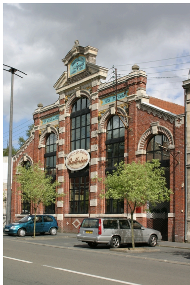
Façade antérieure. Phot. Frédéric Pillet IVR22_20050206016NUCA
