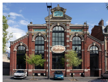
Façade antérieure. Phot. Frédéric Pillet IVR22_20050206009NUCA
