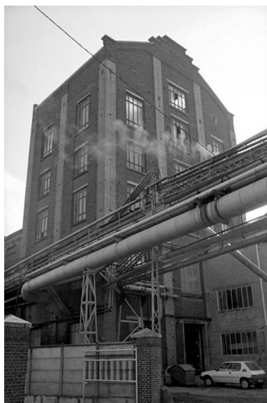
Atelier de fabrication, flanc ouest. Phot. Francis Dubuc IVR22_19908001086Z
