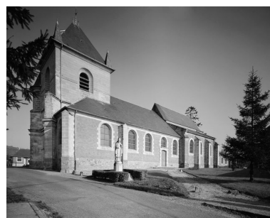
Elévation sud. Phot. Jean-Michel Perrin IVR22_19846001320V
