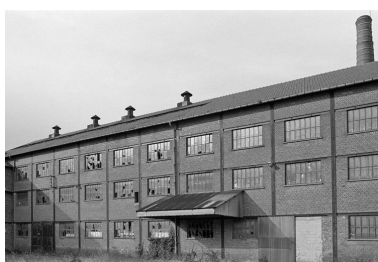
Atelier de fabrication, flanc sud. Phot. Francis Dubuc IVR22_19908001223Z
