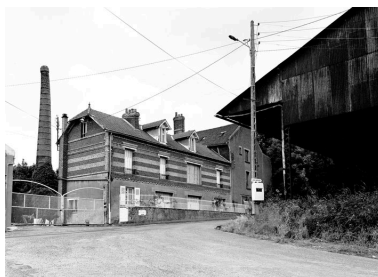
Logement patronal. Phot. Patrick Glotain IVR22_19936000633X
